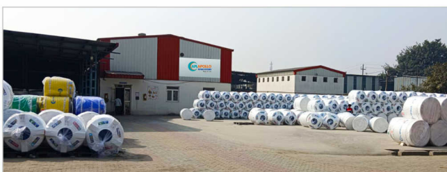
Manufacturing Plant - Sikandrabad (U.P.)
